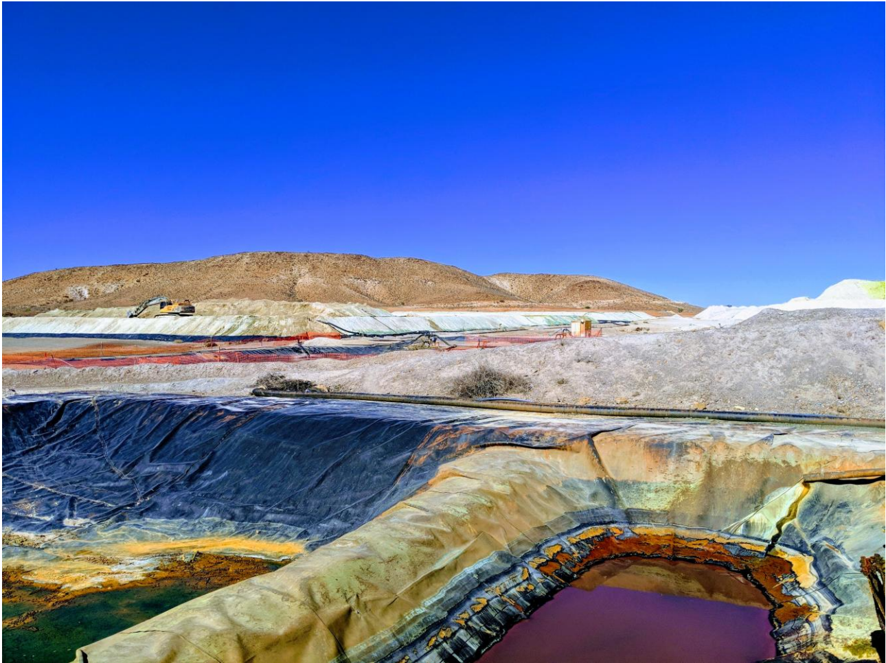
Fig. 6 – Tailings ponds and existing infrastructure
