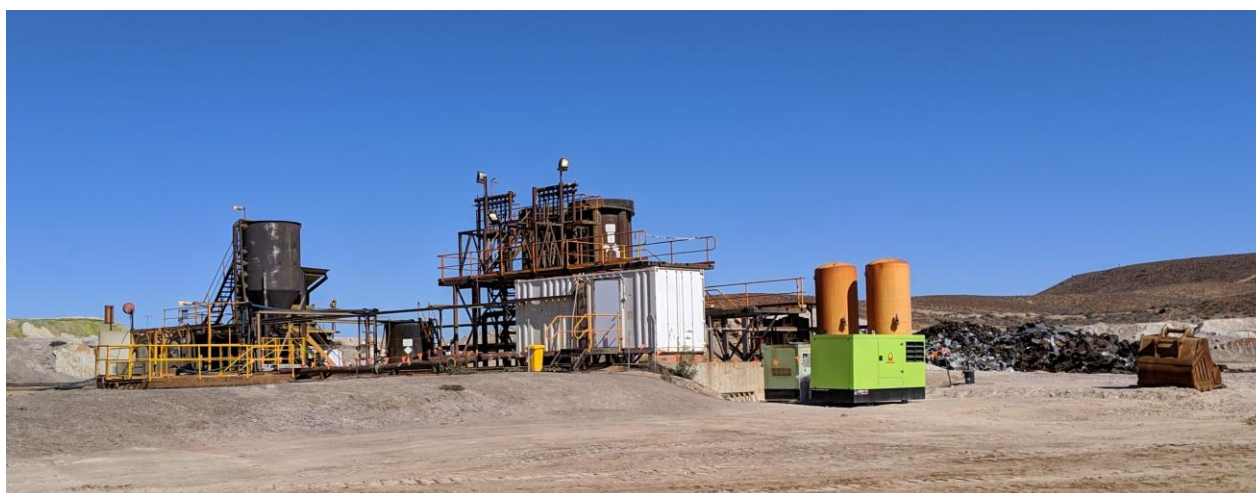
Fig. 7 – Existing mill infrastructure
