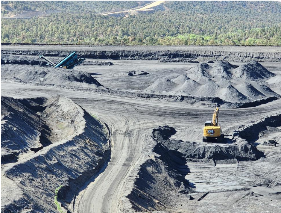
Fig. 3 - View of Cobre resource and open pit under excavation
